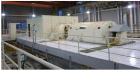
POWER PLANT Capacity : 15 MW Turbine & 2 Boiler x 40 ton
