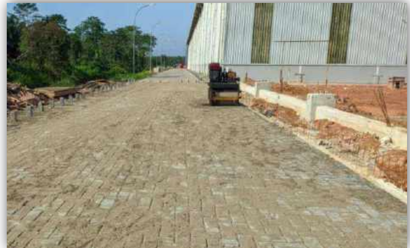
Road Construction Progress
