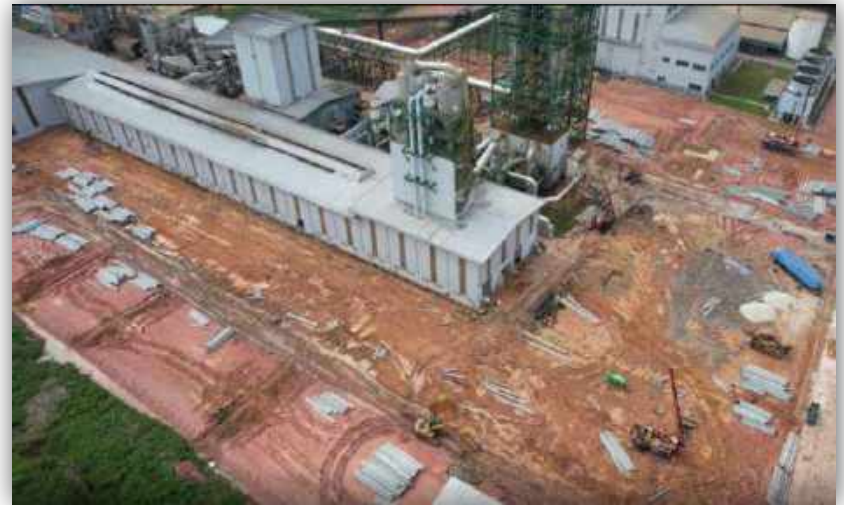
MDF Building – piling stage
