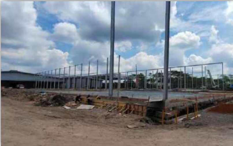
PPIC Warehouse – Structure construction stage
