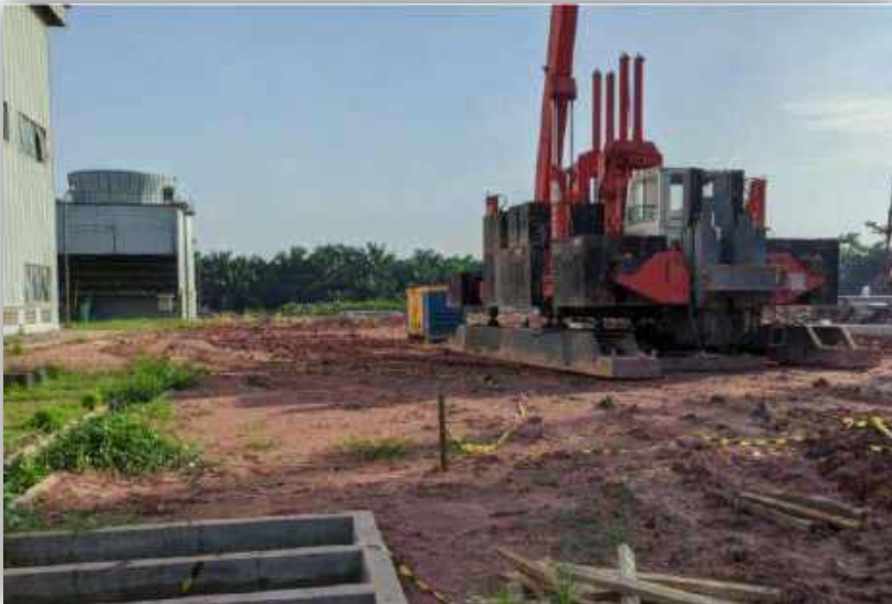
Power Plant Building – piling stage
