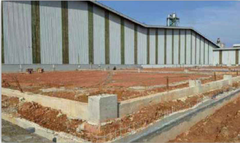
Rawboard Building - pilling stage finished
