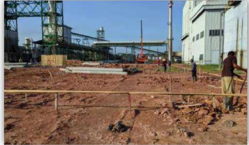
Refiner Building – pilling stage finished
