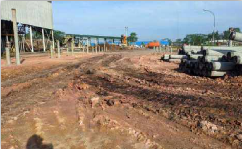
Barker Building – pilling stage
