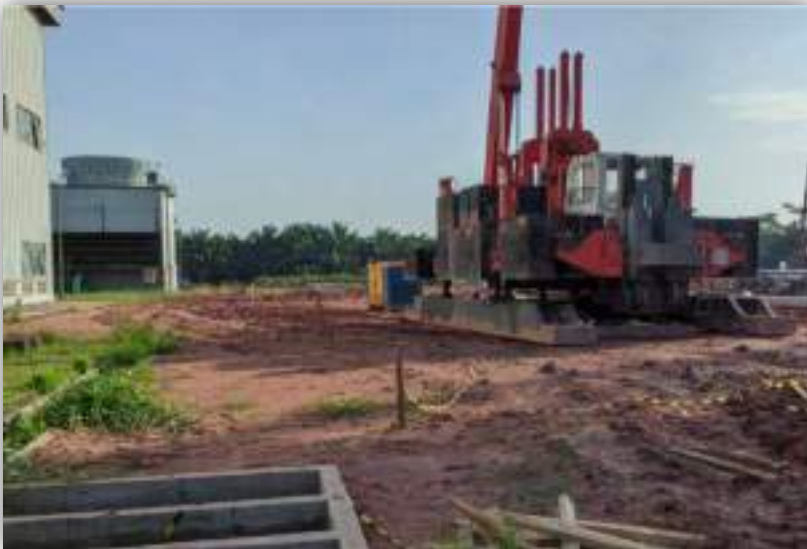
Power Plant Building – tahap pemancangan
