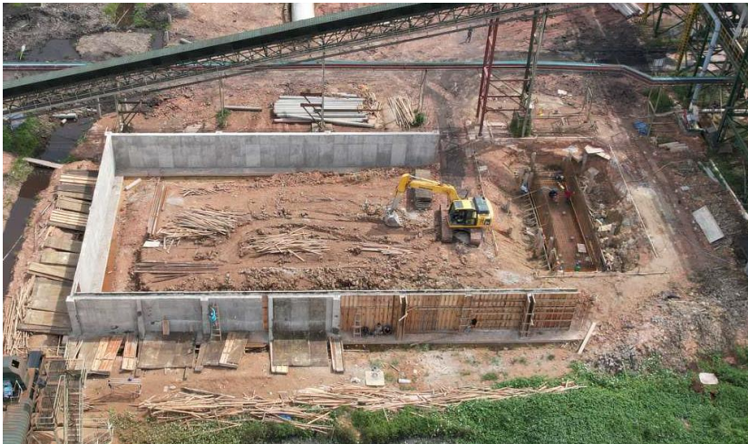
Wet Fuel Building
