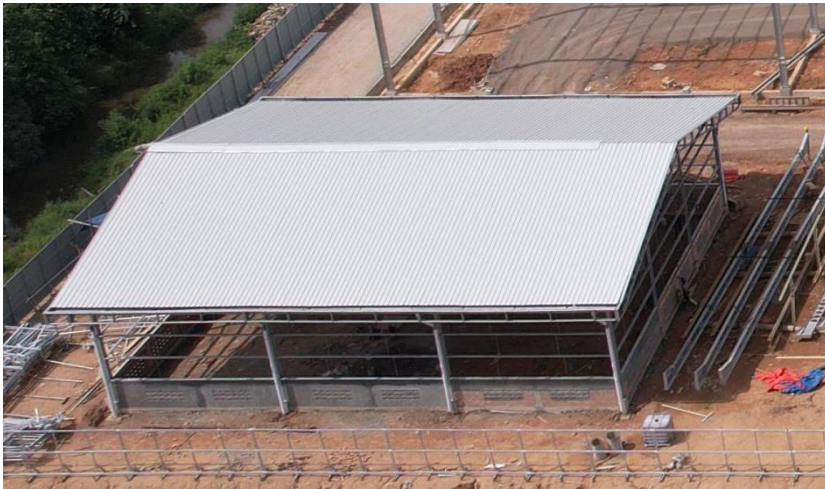
Panel Pallet Building
