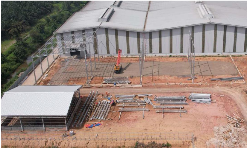
Raw Board Building
