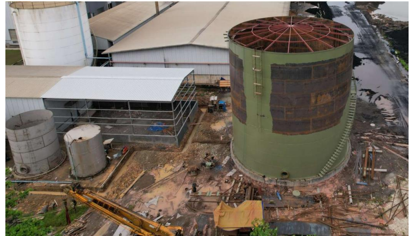
Water Treatment Plant
