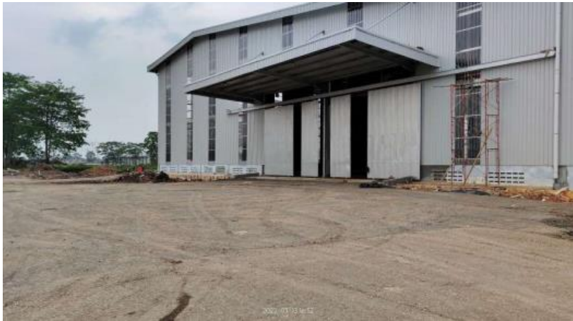
Front view from Jetty
