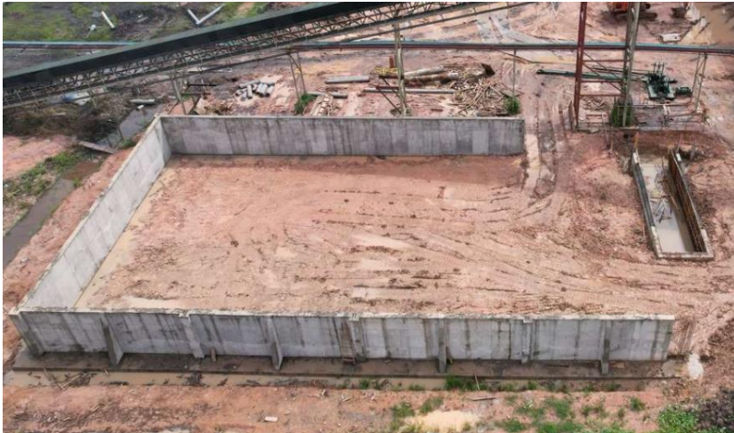
Wet Fuel Building
