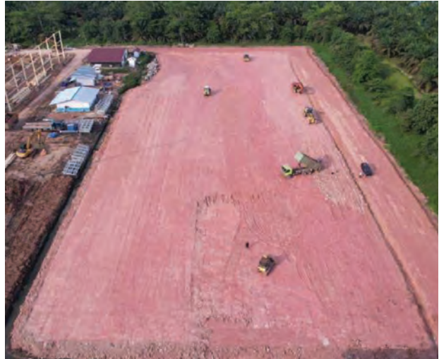
Cut and Fill next to MDF Building
