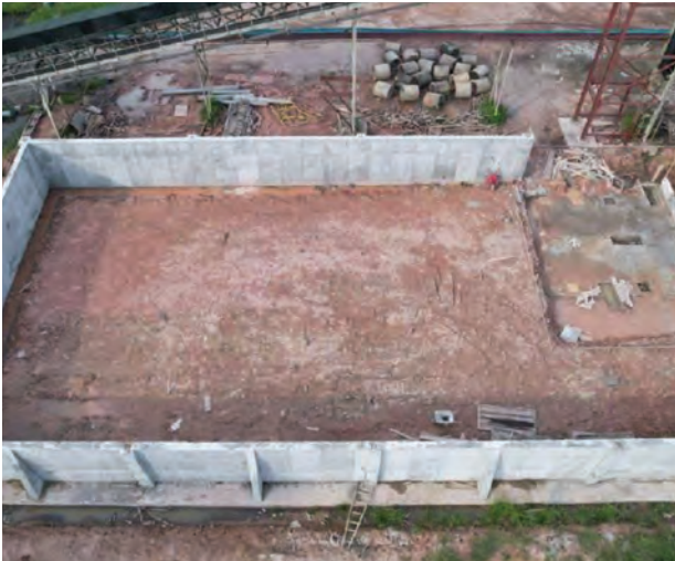
Wet Fuel Building
