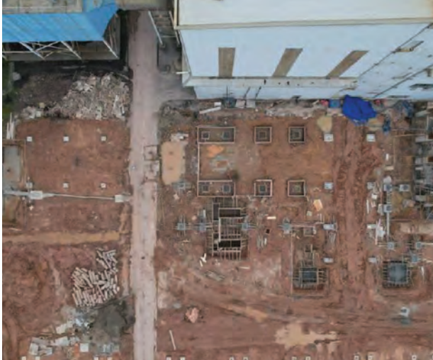
Power Plant Building
