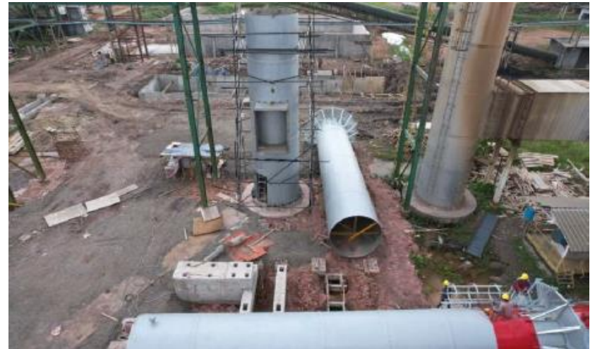
Power Plant – Chimney Erection
