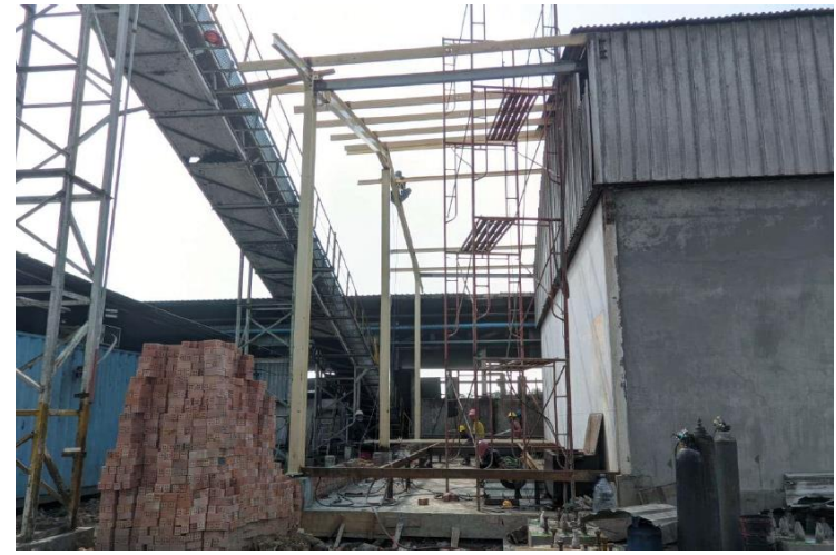
Power Plant – Control Room CHS
