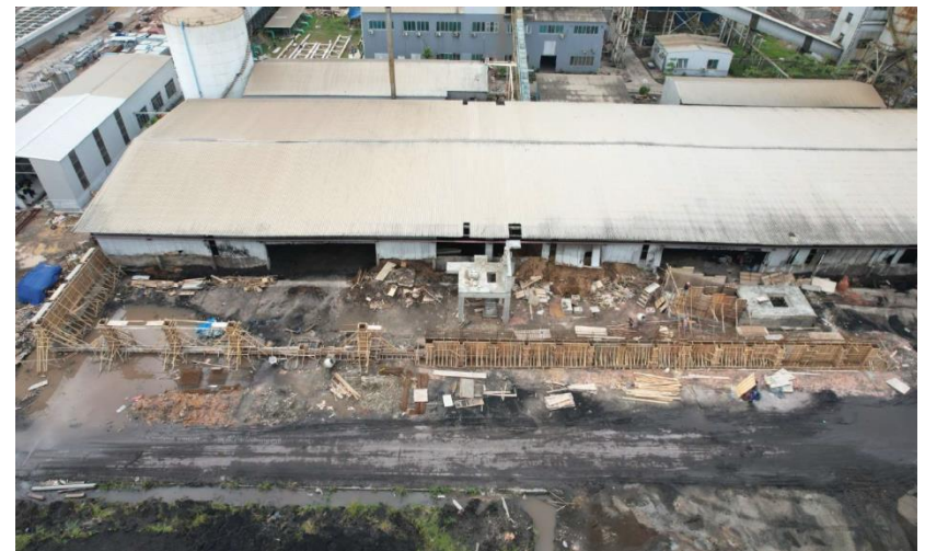
Coal Handling System
