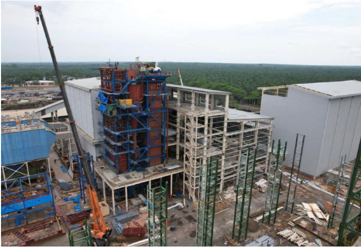
Power Plant – Roofing Process
