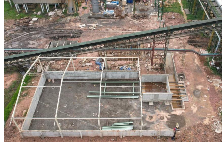
Wet Fuel Building
