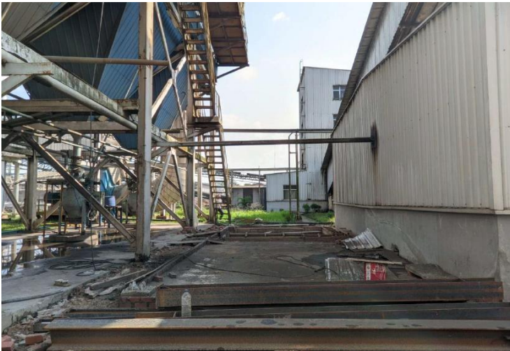
Power Plant – Compressor Room
