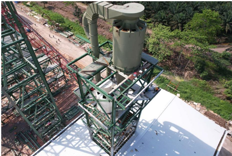
MDF – Forming Line (erection structure)
