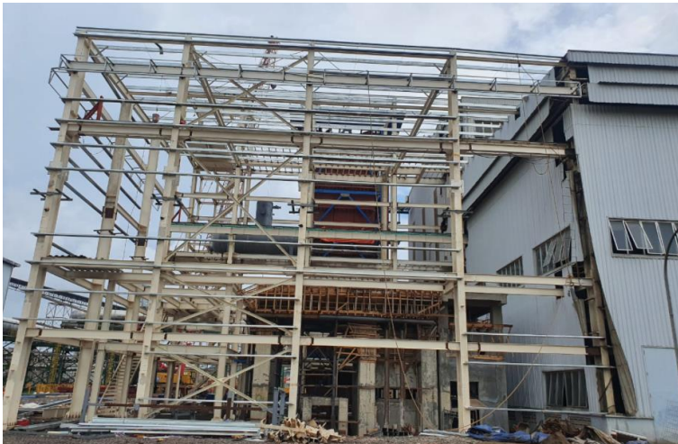
Power Plant – Turbine Civil Work
