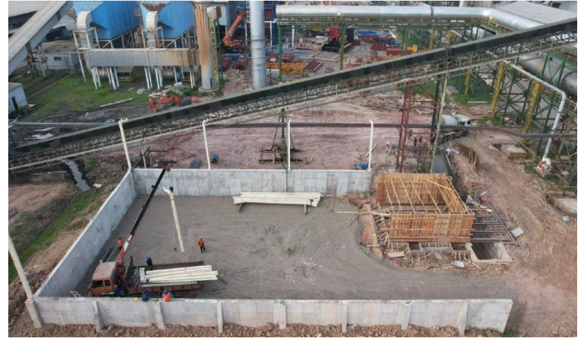
Wet Fuel Building
