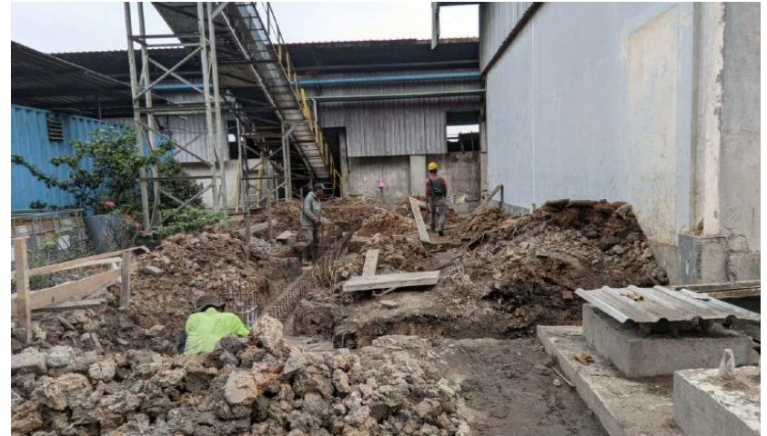
MCC Room CHS
