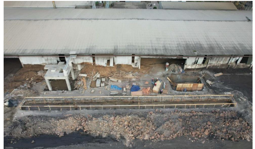
Coal Handling System
