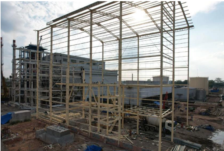
Refiner – On Progress Erection
