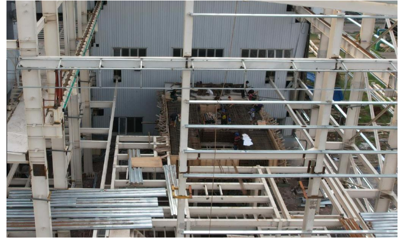
Power Plant – Turbine Civil Work
