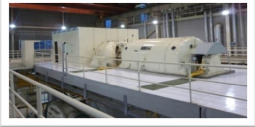
POWER PLANT Kapasitas : 15 MW Turbine & 2 Boiler x 40 ton
