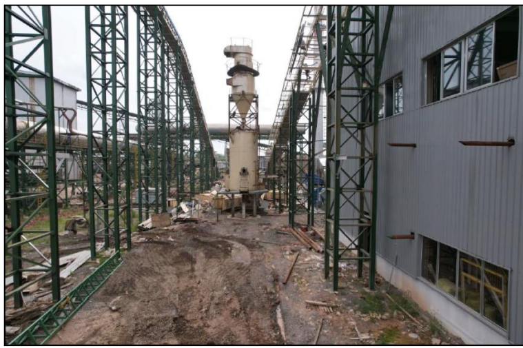
Power Plant – Erection Dust Bin
