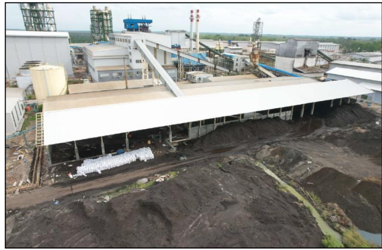
Coal Handling System
