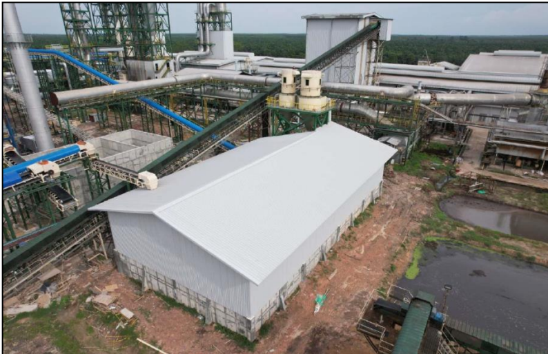
Wet Fuel Building
