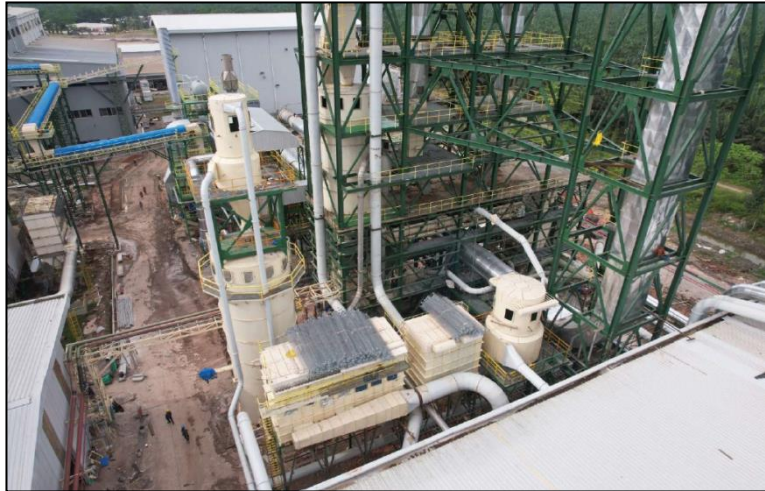
Pneumatic structure and erection dust silo
