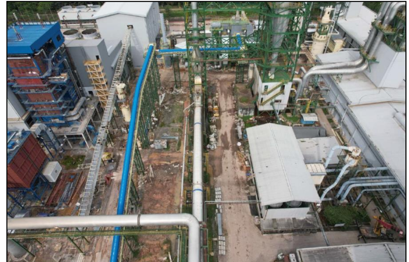
Conveyor Wet Fuel – Energy Plant
