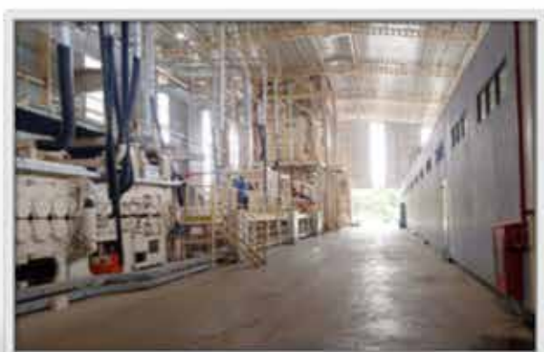
MDF Forming Line with MCC Room Forming
