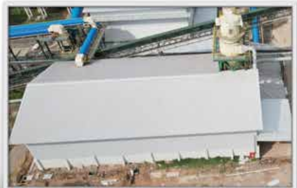
Wet Fuel Building
