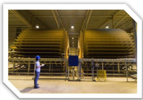
COOLING STACKING & HANDLING SYSTEM
