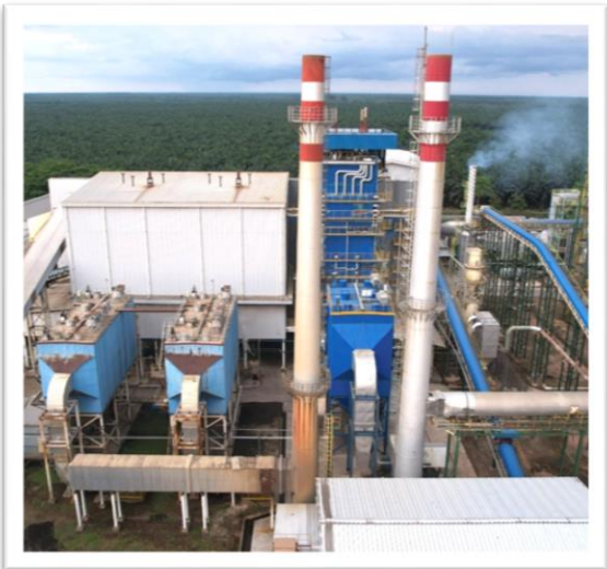
POWER PLANT Capacity : 30 MW Turbine, 2 Boiler x 40 ton & 1 CFB Boiler x 80 ton
