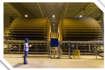
COOLING STACKING & HANDLING SYSTEM
